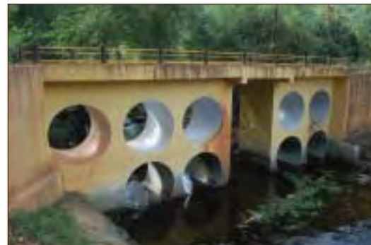
Pipe Bridge - Karuvara
