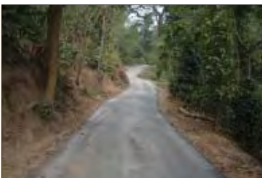
Kattakkad - Puliwara road
